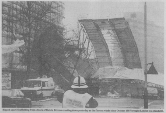
Shipped apart: Scaffolding from a block of flats in Belston crumpled down yesterday as the fiercest winds since October 1987 brought London to a standstill.
